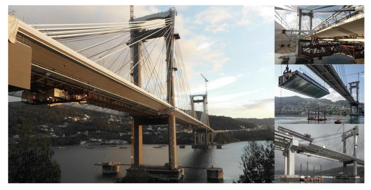
Rande Bridge is a cable-stayed bridge with a 400-meters main span, which crosses Vigo Ria in Pontevedra (Spain) since 1981. The bridge was designed by Italian engineer De Miranda. The existing 694m-long cable-stayed bridge is divided into three spans with lengths: 147m-400m-147m. The existing deck is 23,5m wide.
